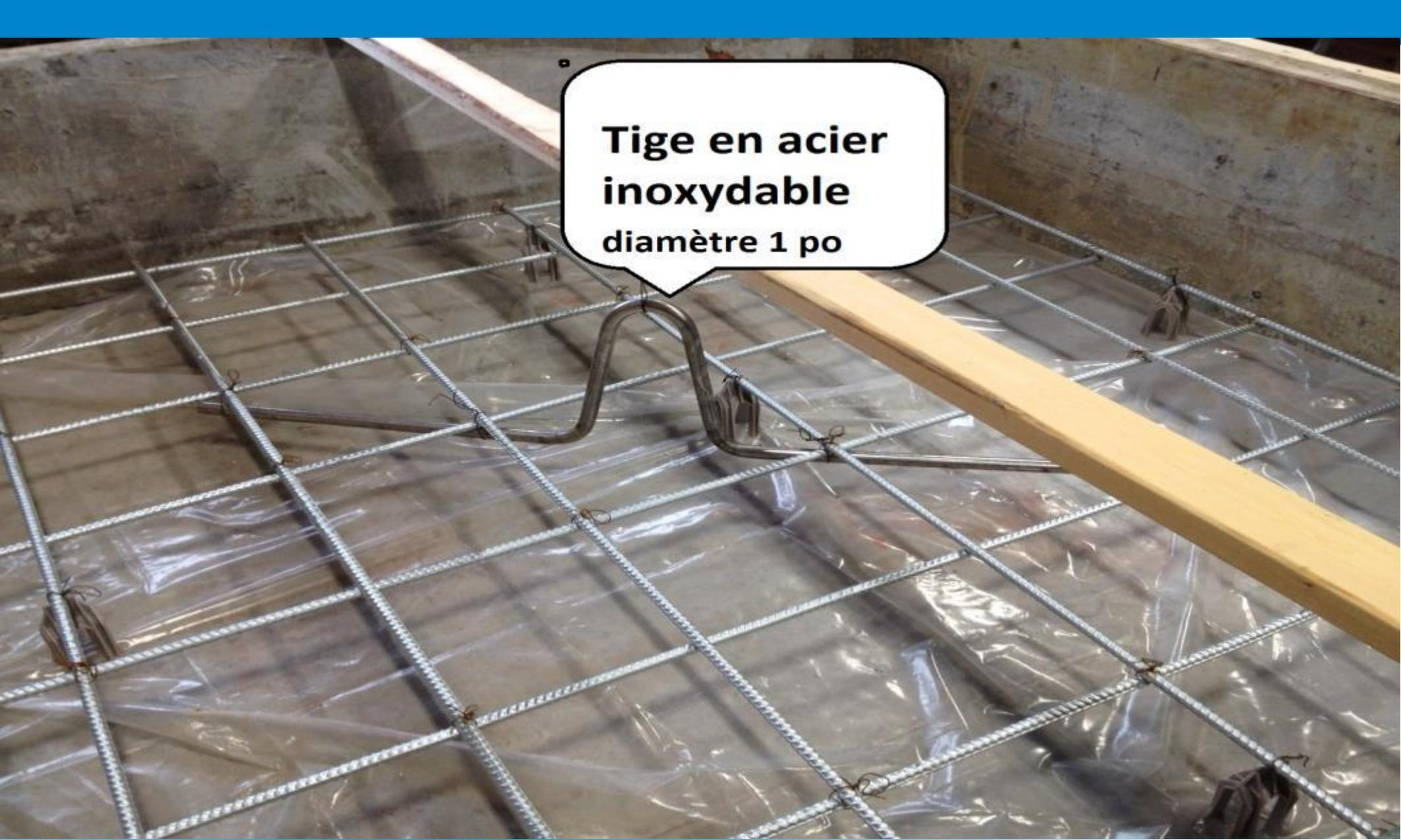
A photograph showing a grid of stainless steel reinforcement bars (rebar) laid out on a concrete slab. The rebar is arranged in a rectangular pattern and is held up by plastic spacers. A wooden beam is visible in the foreground, and a metal hook is attached to one of the rebar. A speech bubble points to the rebar.
